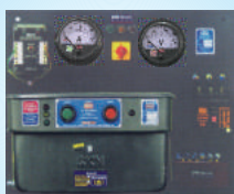
FAB (TPP) CONTROL PANEL
