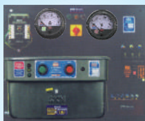
FAB (TPP) CONTROL PANEL
