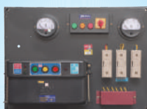
BSA (TPP) CONTROL PANEL
